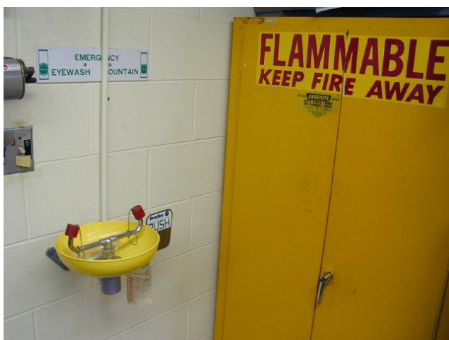
Figure 6.1 – Flammable Storage Cabinet
